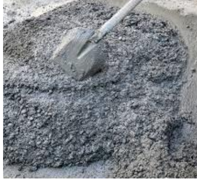
Mixing of concrete
